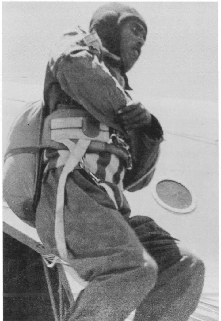
Libyan trooper exits with a D 37. The small pocket on the belly band stows the static line snap hook.
