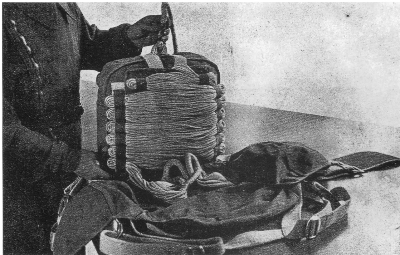
22.) Once completed, the organization of the ropes, place the sack near the shoulder straps and make sure the cord system is facing the bottom of the case.
